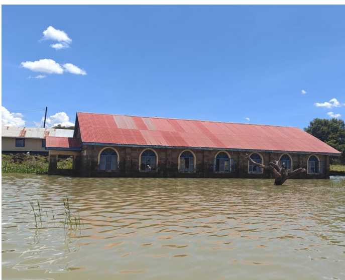
Church affected by Lake Baringo waters rising
